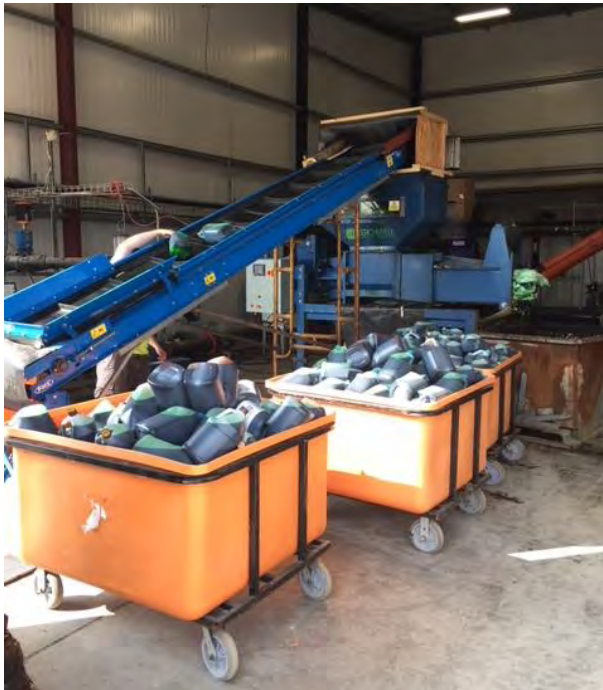
Noblehurst Green Energy, NY
